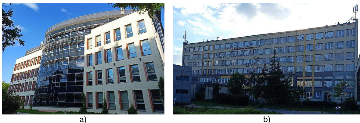
Fig. 1: Educational buildings of Kielce University of Technology: a) "Energis", b) "D" building.
